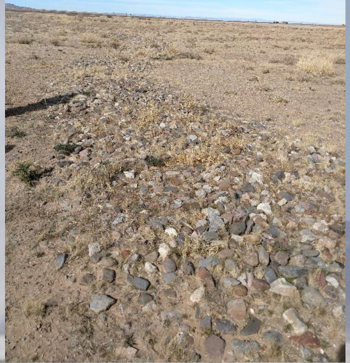
Channel Erosion Area
