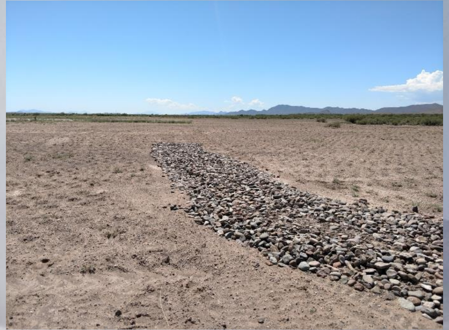
Channel Erosion Area
